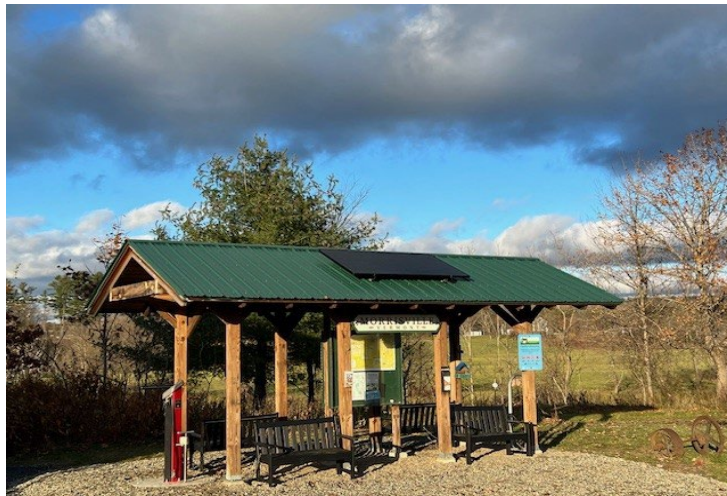
Rail Trail Kiosk Project funded by the Village Special Project Reserve Fund
